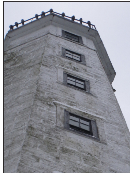
It will cost about $100,000 to scaffold, tent, scrape, and repaint the lighthouse. We also have damage from Superstorm Sandy to fix, including the walkway and sea walls. Over time, we also hope to rebuild the dock. Watch for our fund-raisers or donate at nlmaritimesociety.org .
