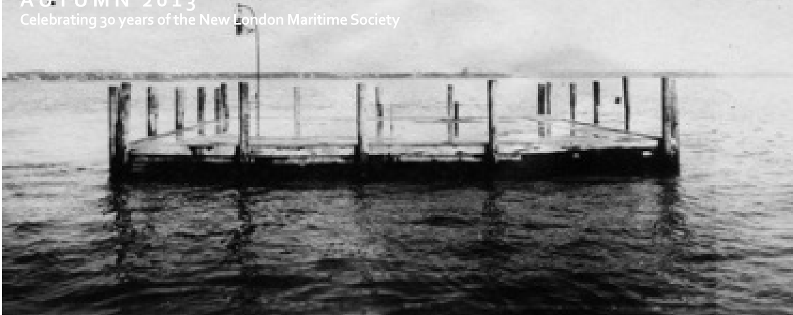
Above: The foundation of New London Ledge Lighthouse, ca. 1908. Photograph courtesy the Henry L. Ferguson Museum Collection.
